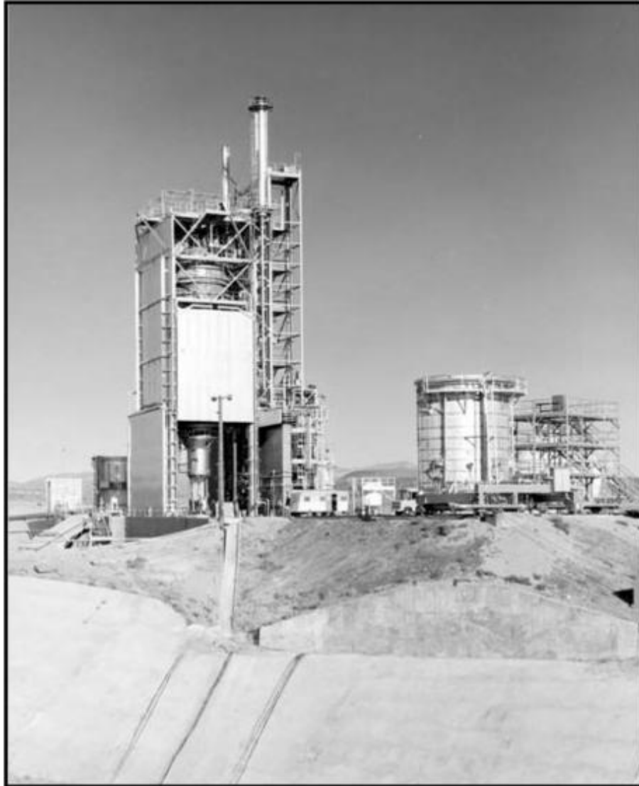
Test Cell C, Nuclear Rocket Test Station, Nevada. Courtesy of the U. S. government.
